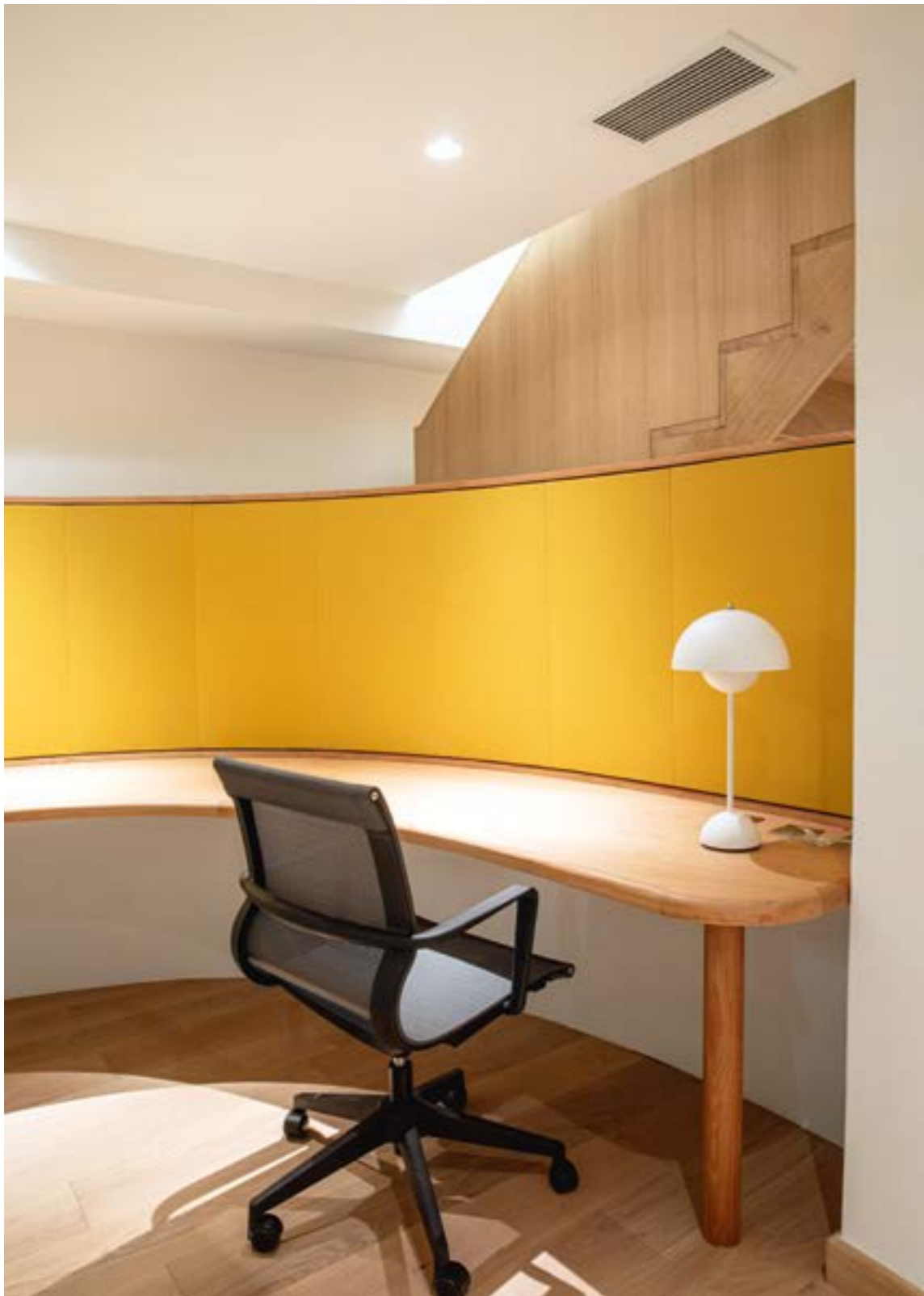
Vibrasto acoustic cladding applied to curved permanent fixtures in Cerfrance accountants' offices in Paris. Interior designer: Capucine Beauamps of Wrk, 2021.
