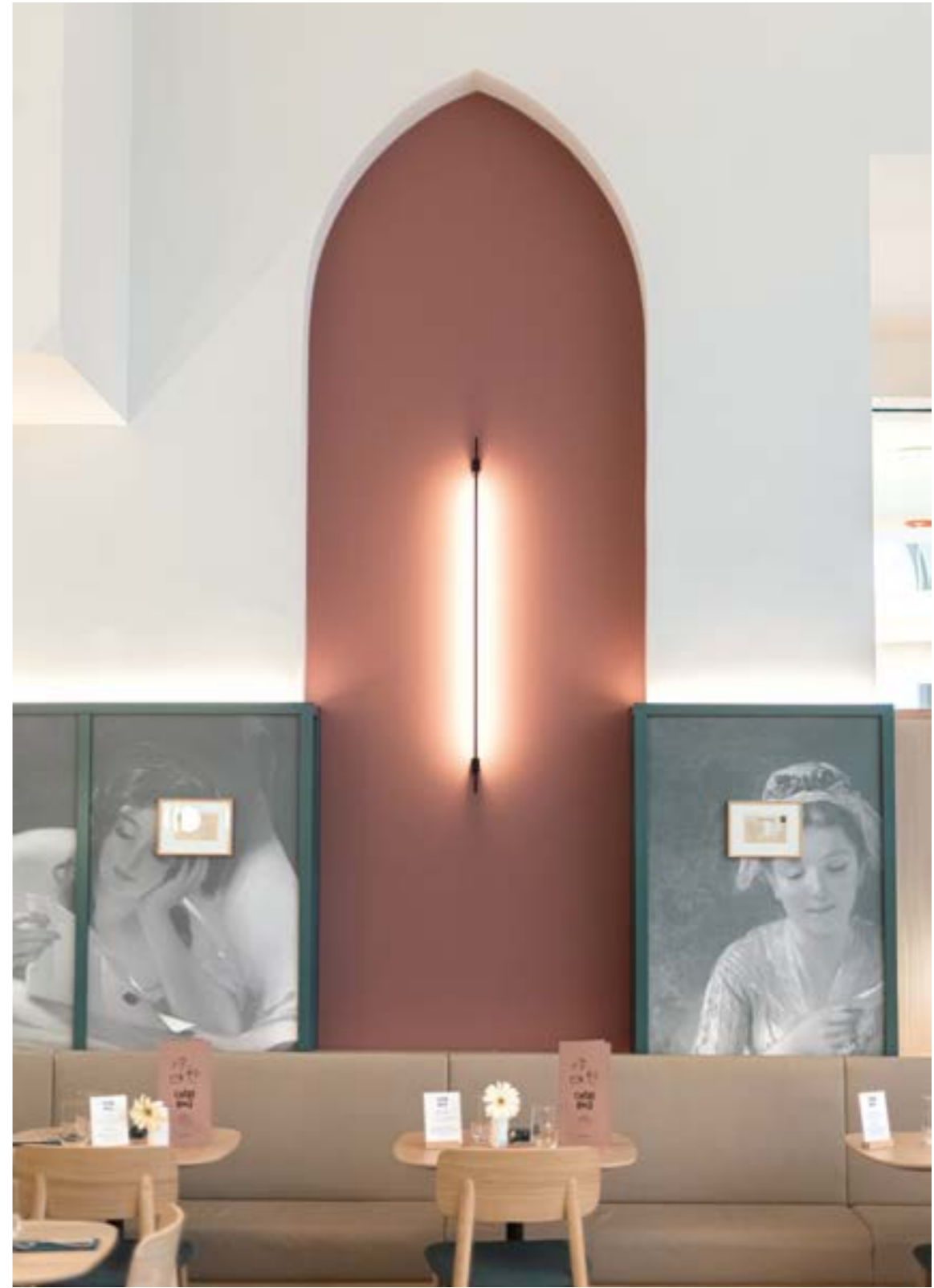
Vibrasto acoustic cladding installed in an alcove. The flexibility of the tensioning battens makes it possible to fit the shape. The Chère Amie restaurant in Strasbourg. Design: Pascal Claude Drach, 2023.
