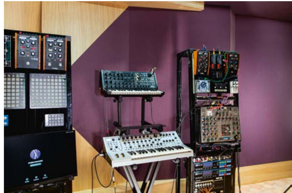
Vibrasto acoustic cladding on the wall of Bordeaux recording studio Universeul. A custom-made heather designed by Christian Malcurt was installed for recordings by the band Odezenne.
