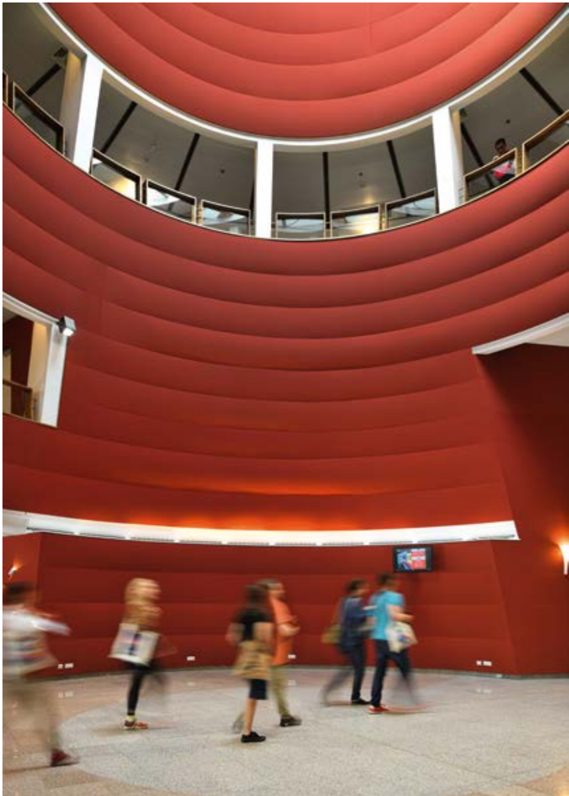
Vibrasto acoustic cladding fitted to a wall in the Polydome Congress Centre in Clermont-Ferrand in central France. Yves Bellaigues, Clermont-Ferrand city architect, 2022.
