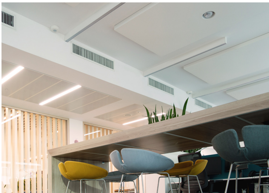
MILANO Architect Progetto CMR Realization Progetto Design & Build
